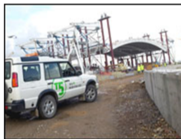
Construction at the terminal is well underway
